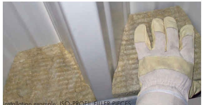
Installation example: ISO-PROFIL FILLER PIECES
