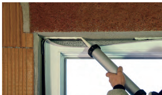
Installation example: ISO-TOP FLEX-ADHESIVE SP
