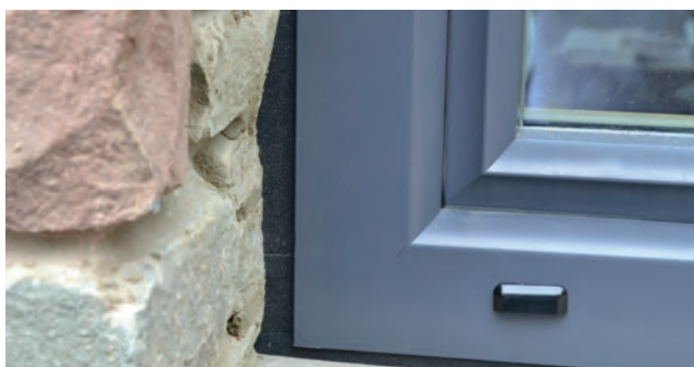
Installation example: ISO-BLOCO AIR
