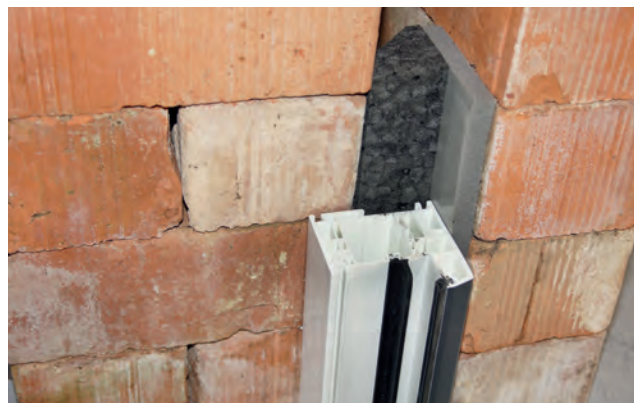
Installation example: ISO-BLOCO FILLER
